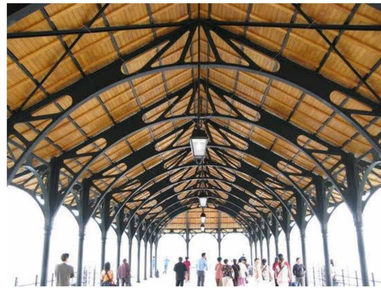
CASE STUDY - BLAKE PIER - HONG KONG, CHINA
